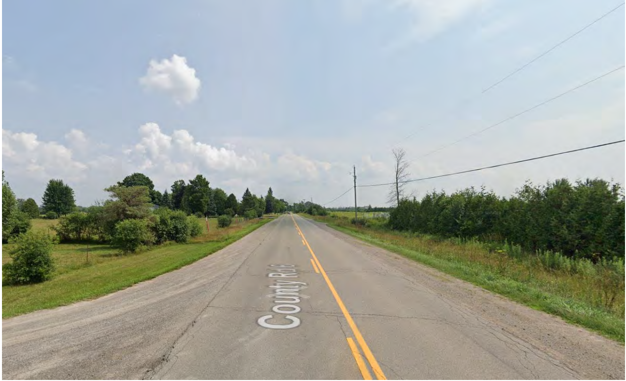
Figure 4 Site context, looking south towards Rows Corners Intersection
